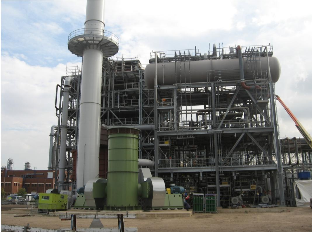
Industrial Boilers are direct-fired boilers designed and used to provide steam to industrial processes. They may use various type of fuels, liquid or gaseous, according to the application. An Industrial Boiler is generally made up of two major systems. One system is the fuel-air-flue gas system (fireside) and the other is the water-steam system (waterside). Heat is provided to convert water into steam.
